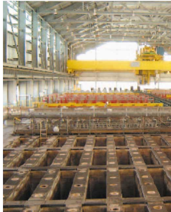
Sohar Aluminium Baking Furnace (courtesy of Sohar Aluminium)
