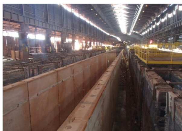
Central casing wall replacement
